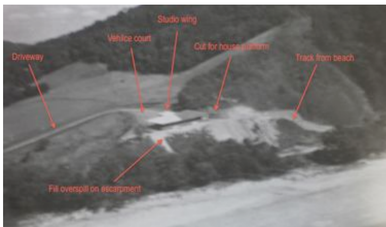
Fig 25. Aerial view c1960/61 (Peter Kellett). Note, to form a building platform, Busst has cut selective trees (as seen in Fig 21); excavated dirt has been pushed over the pre-existing embankment and a cut has been formed into the hillside to the north to form the track to the beach. Note also re-growth over the previously cleared hillside north of the house indicated by change in tone and texture.
